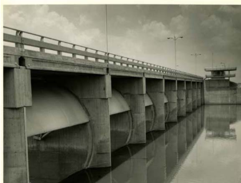
"Pearl River Reservoir Spillway, showing the gate system of control" June 1963 from the Hugh W. Shankle Collection, Mississippi Department of Archives and History
